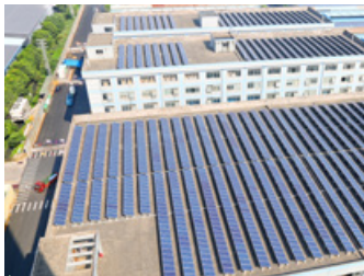
Solar power generation on the rooftop of the headquarters 總部屋頂太陽能發電
